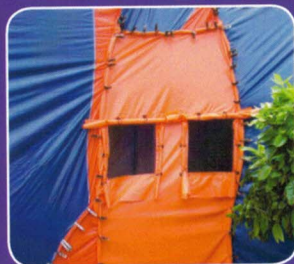
Example of fresh air intake inlets
