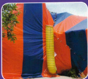
Example of duct
